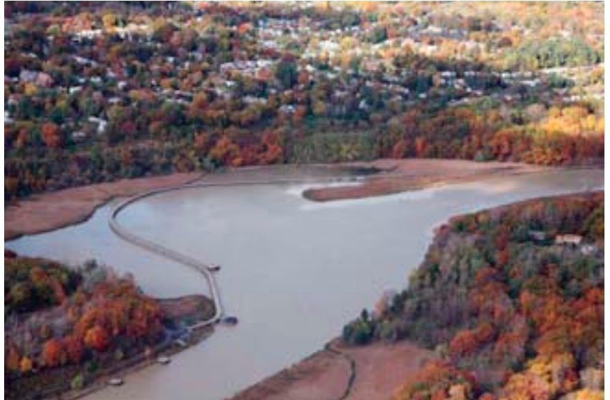
An 86-span, 3,572-foot-long pedestrian bridge helps complete the 15-mile Genesee Riverway Trail near Rochester, N.Y.
